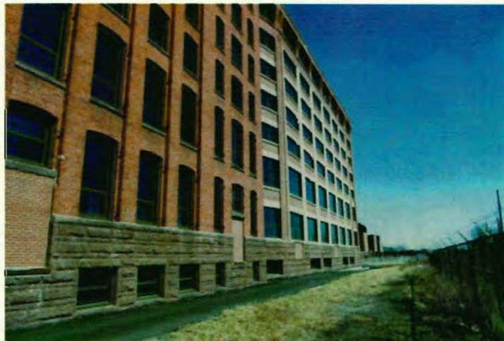
Variety of window types and sizes evident in this view of the south elevation of the Stanley Building.
