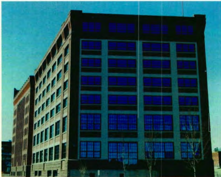
East view of Stanley Building
